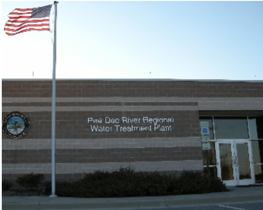
Figure 6-28. City of Florence Surface Water Treatment Plant.
