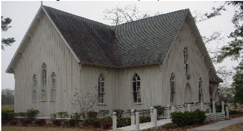
Picture courtesy of Florence County Planning Department staff: March 15, 2007
